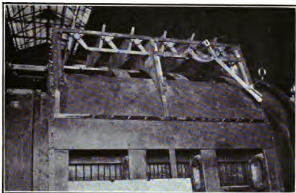
FIG. 84.—U. S. S. California : View of Alternator Showing Air Discharge Damper
